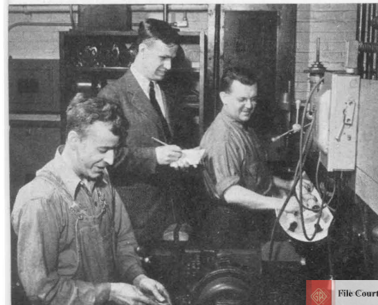
The standardizing laboratory is under the direction of W. G. Webster, Engineer ( left ), and M. C. Hobart, foreman ( right ). Great responsibility rests with this department, which performs the final test and inspection on all instruments.
