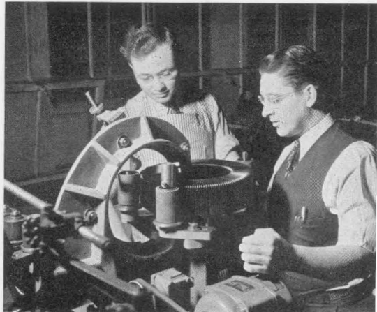
One of the jobs of the winding and transformer assembly department is to produce Variacs. C. W. Whitehead (left) operates the machine winding a TYPE 50 Variac. At the right is R. W. Searle, foreman.
