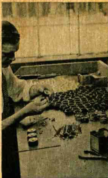
9 - ASSEMBLING SLIDE WIRE ATTENUATORS
