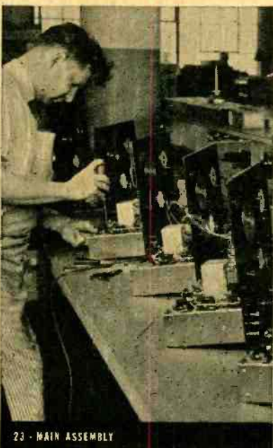
20 - ASSEMBLING OSCILLATOR SHELVES
