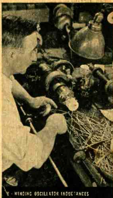
7 - WINDING OSCILLATOR INDUCTANCES
