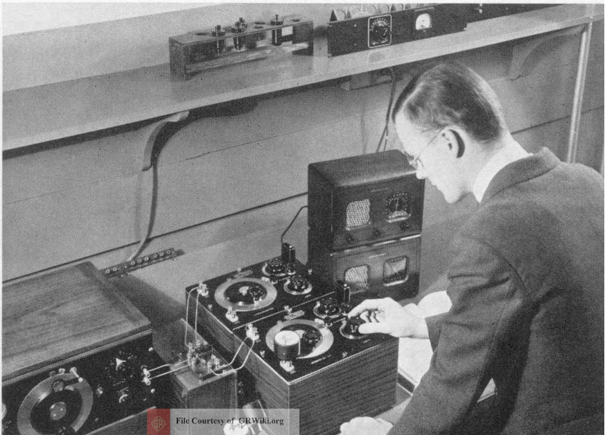
FIGURE 1. Two TYPE 721-A Coil Comparators arranged for testing coils at two frequencies.
