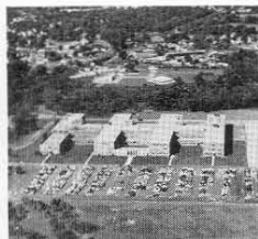
Airplane view of the new General Radio Plant.
